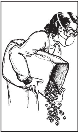
Figure 2: Wear protective clothing when installing insulation.
